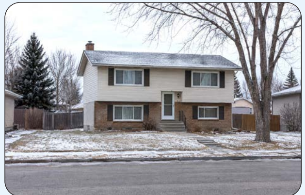
Figure x.5 - Regina's 1977 conservation house needed no furnace at all. Thick walls and a sealed shell kept the cold prairie air from getting inside.
