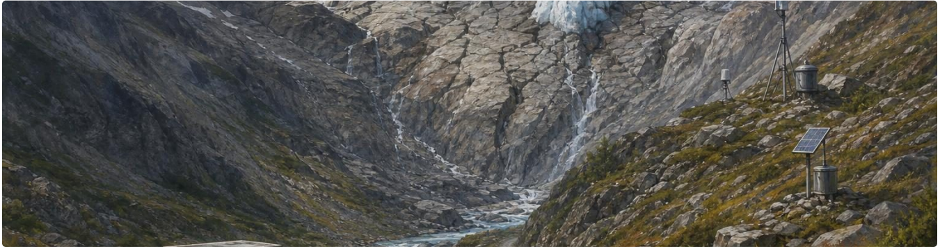
A mountain valley with infrastructure below a retreating glacier and cracked rock slope, with monitoring equipment in place.
