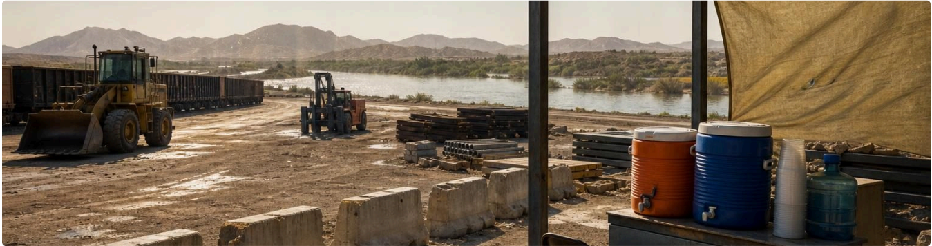
An empty freight and utility worksite sits beside a low river under intense heat, suggesting drought, transport delays, and jobsite safety concerns.
