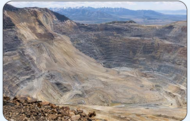
Figure x.5 - Bingham Canyon Mine shows how far a landslide can travel. Ground sensors gave workers enough warning to evacuate hours before the slope gave way.
